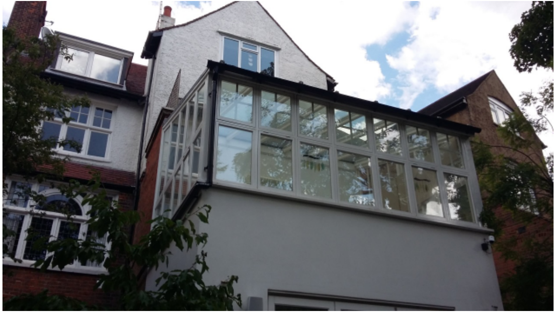
View of existing rear extension
