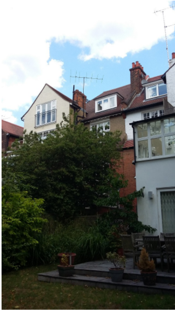
View looking to attached house to North-West
